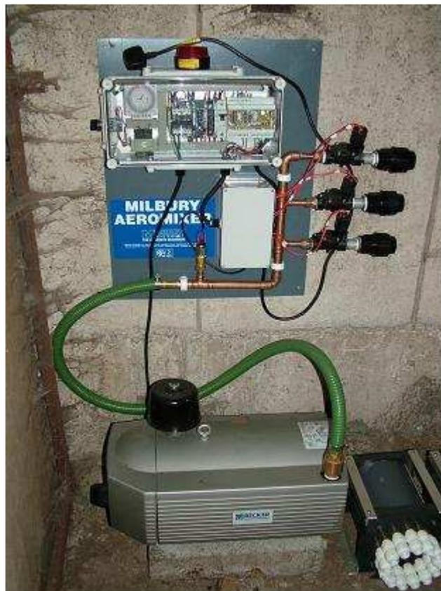
**Figure 5** Air compressor, control panel, manifold and rotary valve of aeration system
