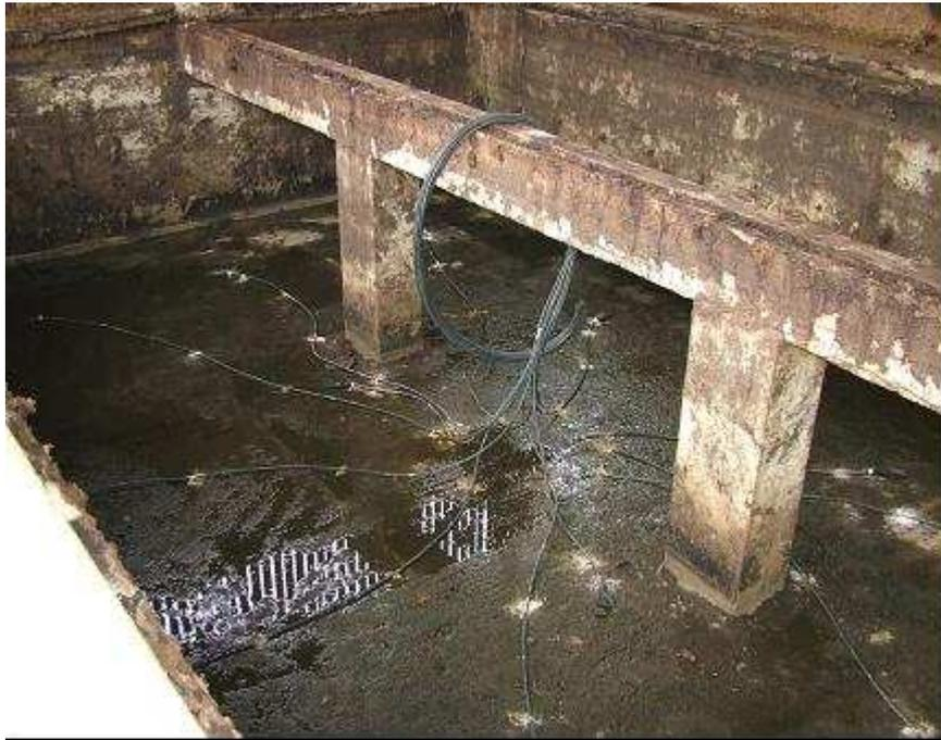
**Figure 4** Installation of air delivery nozzle system into slurry tank
